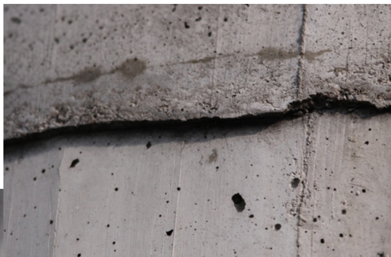
Offset of plane – horizontal joint.
