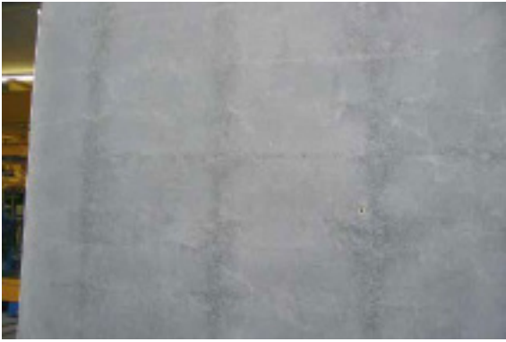
Fig. 5.3 Imprinting of the reinforcement
